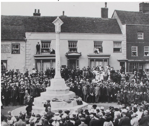
The surviving shopfront of the former Gammer's Stores, seen on the occasion of the dedication of the War Memorial in 1921
